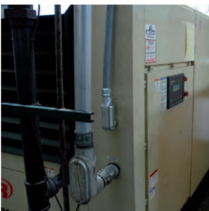
Air Compressor Control
