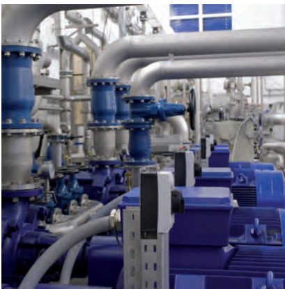
Industrial Pump Control
